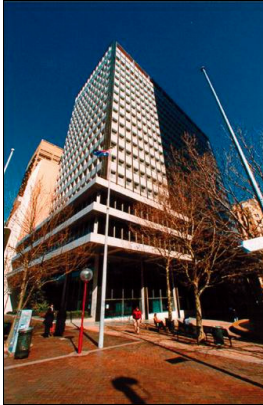
Reserve Bank Building 4,000 sqm
